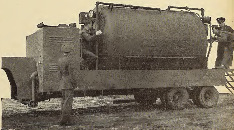
Portable decompression chambers mounted on trailers can be taken right to the front-line airfields to test flying personnel for high altitude operations.
